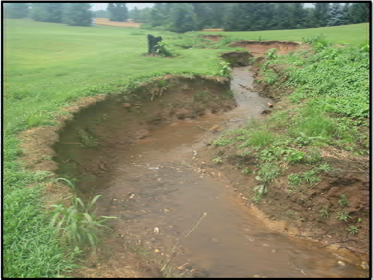
Lack of vegetation contributes to stream bank erosion and scouring.
