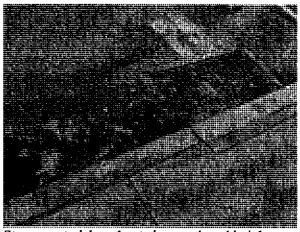
Stucco material washout along curb and in inlet.
