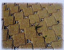
Pavement blocks allow precipitation to infiltrate into groundwater supplies rather than runoff
