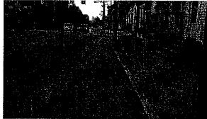
Sediment from sidewalk excavation on roadway.
