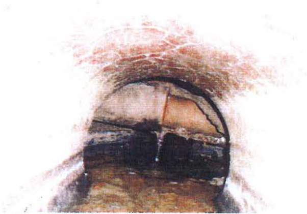
- From SWS Manhole: looking North into 12" SWS pipe to broken lateral.
