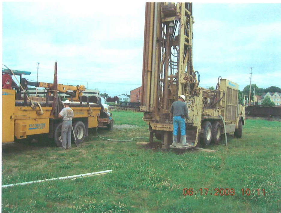
Installing MW-3S.
