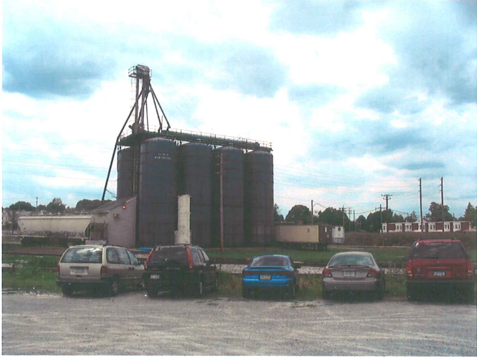
Site looking northwest.
