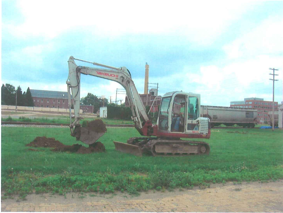
Using Mini-Excavator to check for underground storage tanks.
