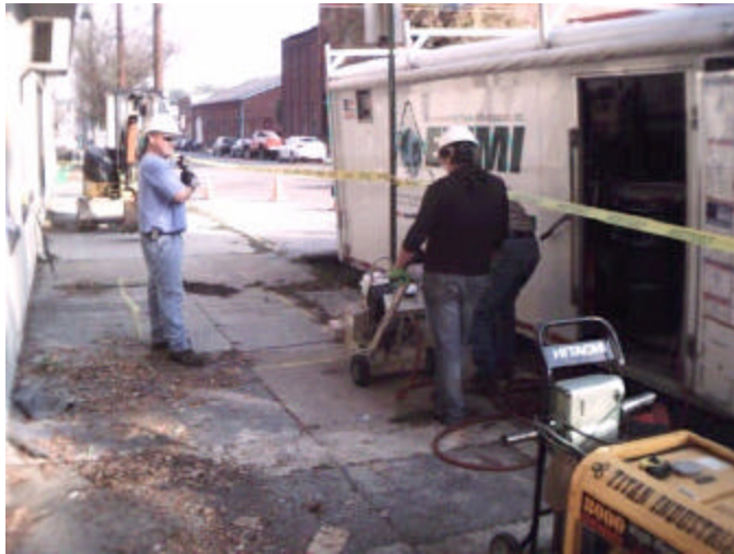
1. Before UST Removal
