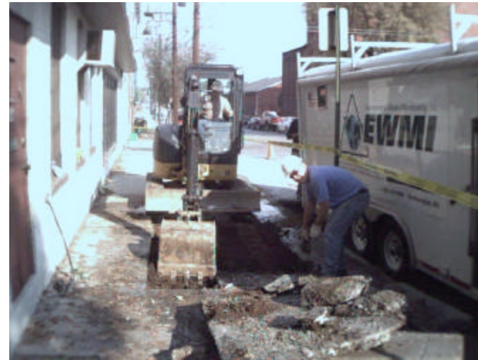
2. Removal of Sidewalk
