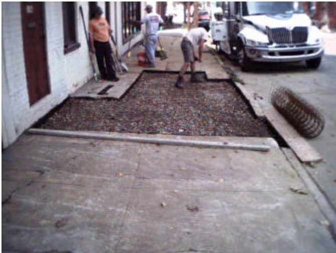
7. Backfilled Excavation
