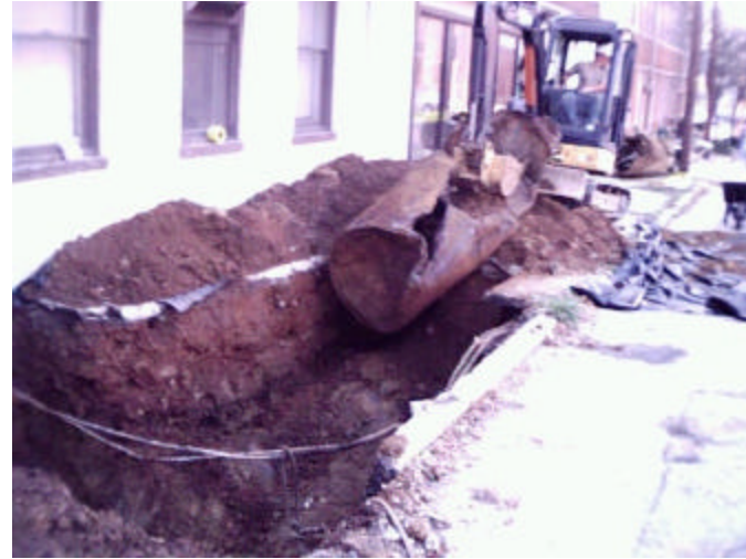
6. Removal of UST 2
