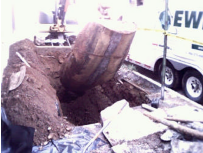
5. Removal of UST 1
